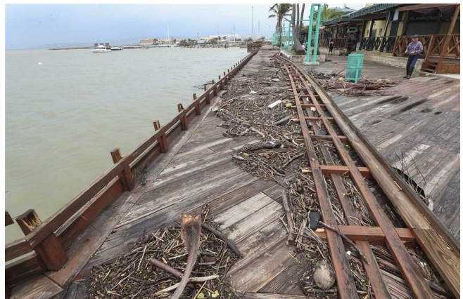
Right: The same pier after this Fall's hurricanes.
